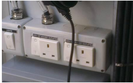
Figure 11: 220VAC Plug Points
