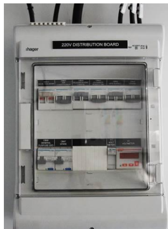
Figure 12: Sub- Distribution of 220VAC Consumers
