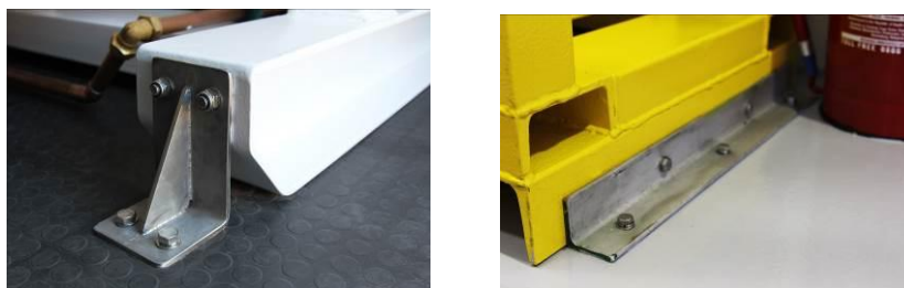
Figure 4: Typical Mechanical Fastening
